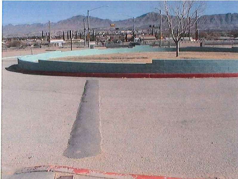
Figure 14 - Riverside ES Main Circle Drive
