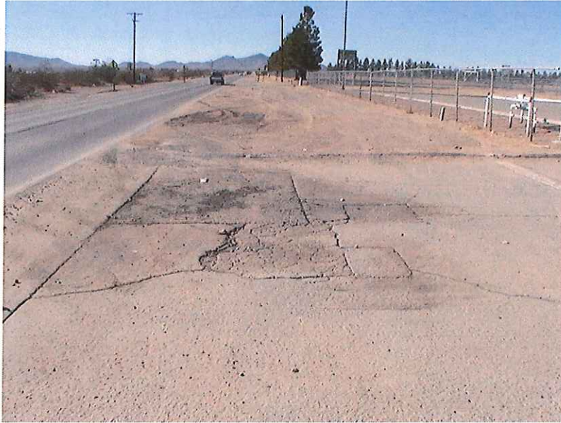
Figure 19 - Chaparral ES Main Parking Entrance
