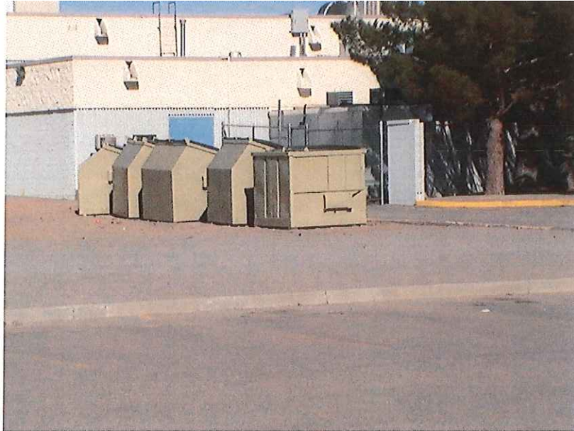
Figure 24 - Chaparral ES Dumpster Area
