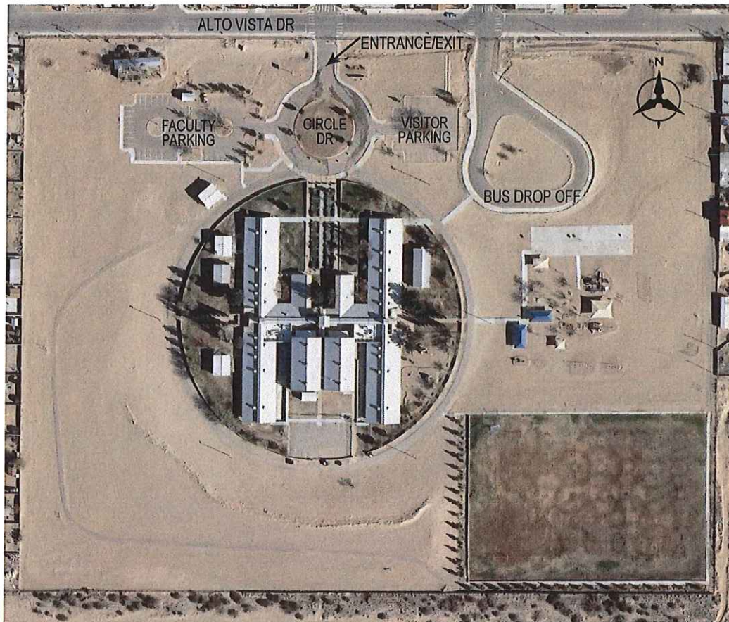
Figure 7 – Sunland Park Elementary School
