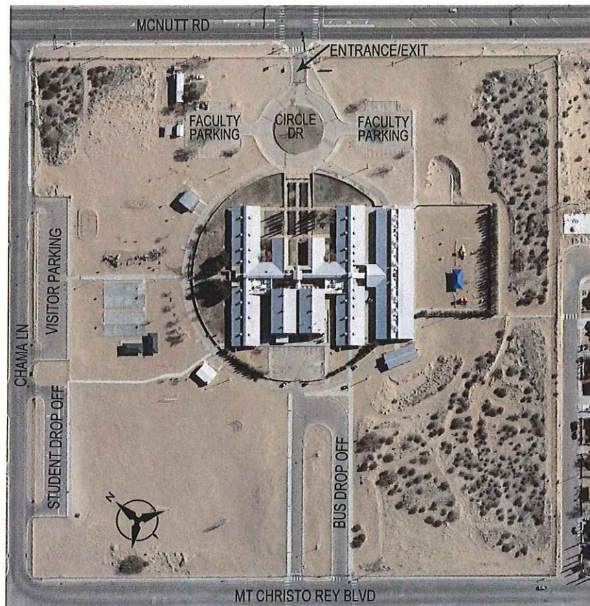
Figure 13 – Riverside Elementary School
