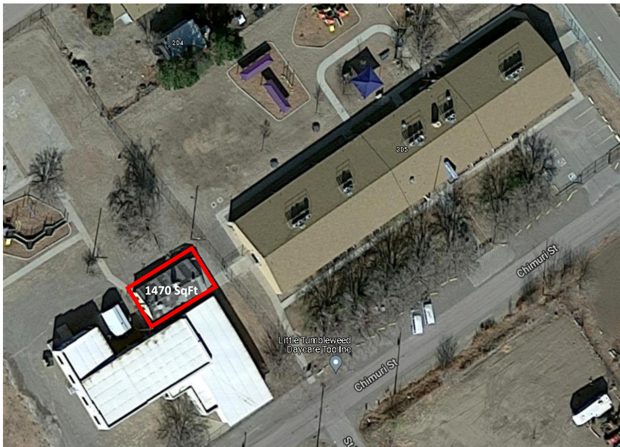
253 E. Chimuri St., La Mesa, NM, black and gray roof storage
